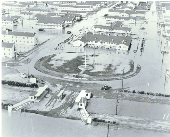
Flooded Front Gate
