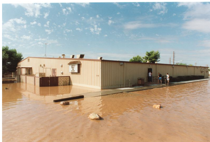
Flooded Base Bowling Alley, 20 October 1992
